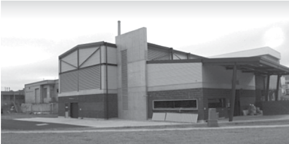
The new ANSTO Health building
